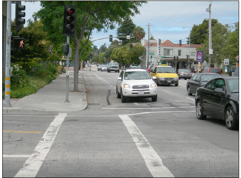
This curb ramp at Laurel @ Front in Santa Cruz places a pedestrian in a wheelchair in the travel lane when they come down the ramp.
