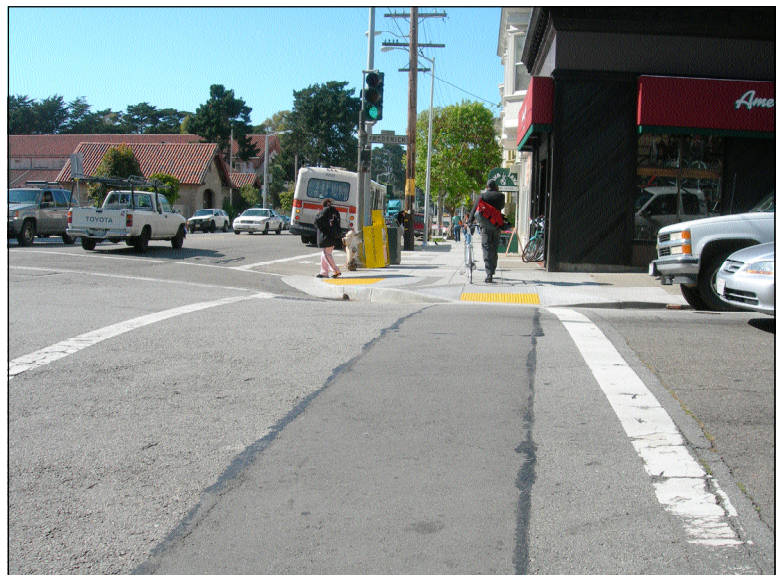
This intersection in San Francisco uses two directional curb ramps.
